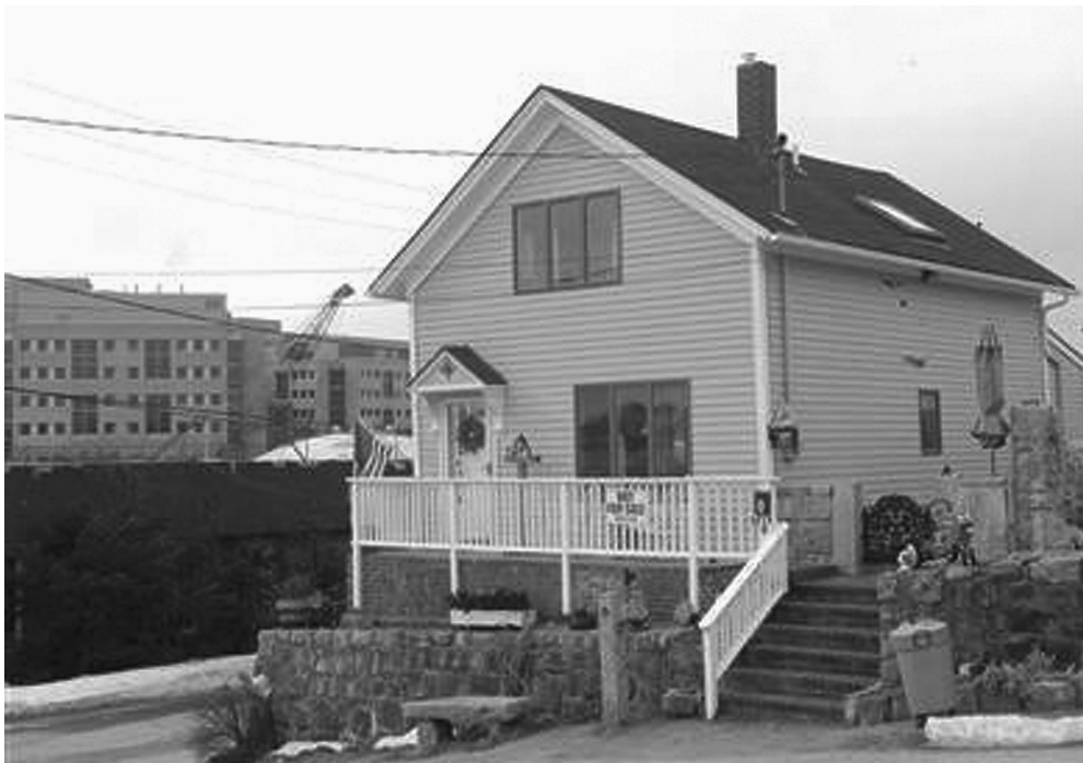
Figure 35.5 Exterior of Kelo home, New London, Connecticut. Center for the Defense of Free Enterprise: Property Rights
