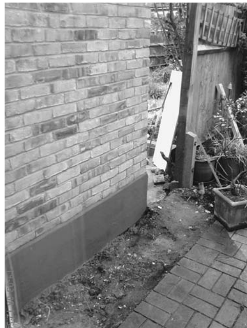
Figure 13.14 The builders next door have almost finished doing stuff on our side of the fence. This morning they rendered the bottom part of the wall. It is still wet. It's sad I have to be careful about photographing while they still are around, because they could see this as criticism of their work (and in the back of my mind looms the nightmare spectre of a court case...). In fact, we're not critical of their work at all. And we like them a lot. I just want to record that the rendering was done today. And it's been done well. But try telling them what's behind taking the photo, and there you come abruptly up against the difference between working- and middle-class cultures. I've been that way before. The look of incredulity. The struggle to bridge the gap
